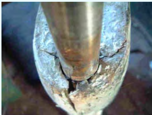
Serious cracking at rudder stock entry
