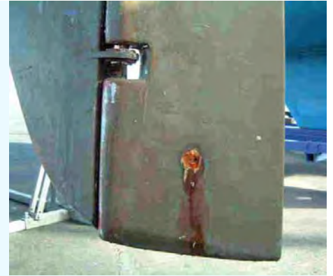
Might be worth investigating the cause of the rust staining
