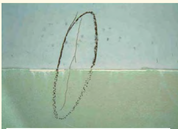
Longitudinal crack in gel coat on waterline. This should be further examined
