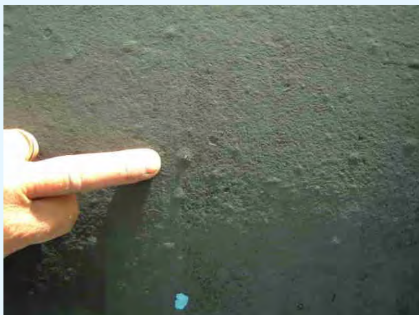
Moderate blistering, these average about 8mm dia, but can be as large as 13mm in advanced cases
