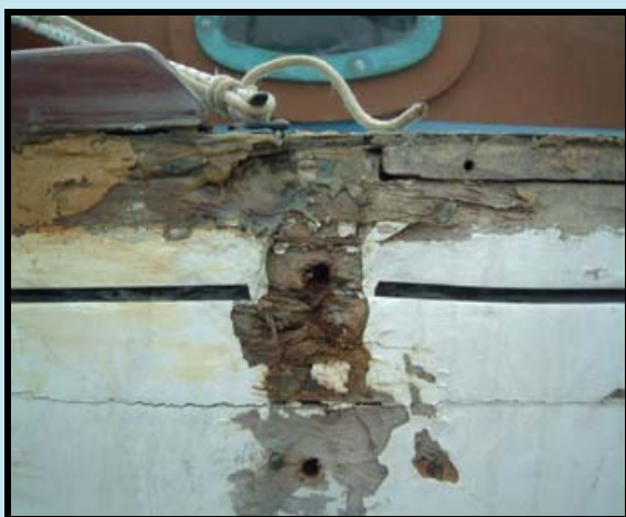
Decay under chainplate extending into deck
