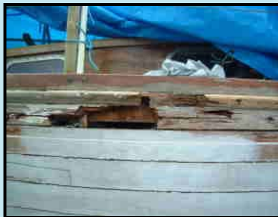
Major sheerplank decay caused by leaking deck
