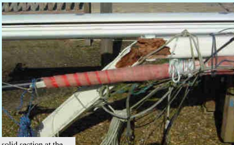
This is a hollow mast but a solid section at the bottom has been compromised over many years by water penetration. The white paint has obscured the continuing deterioration until it broke upon removal for survey
