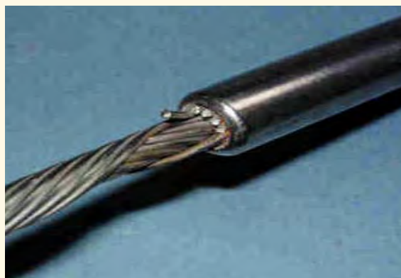
Work hardened & fractured stainless wires at the swage
